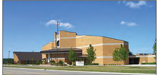
The Auch Company first completed a project for St. Peters Lutheran Church in 1912. In 2006 Auch built the congregations new sanctuary in Macomb, Michigan.
