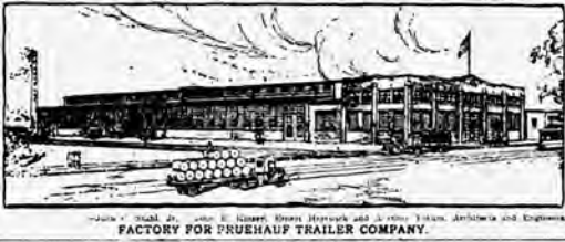
The carpentry contract for the Fruehauf factory was one of the firm's few projects during the building slowdown of the First World War.
